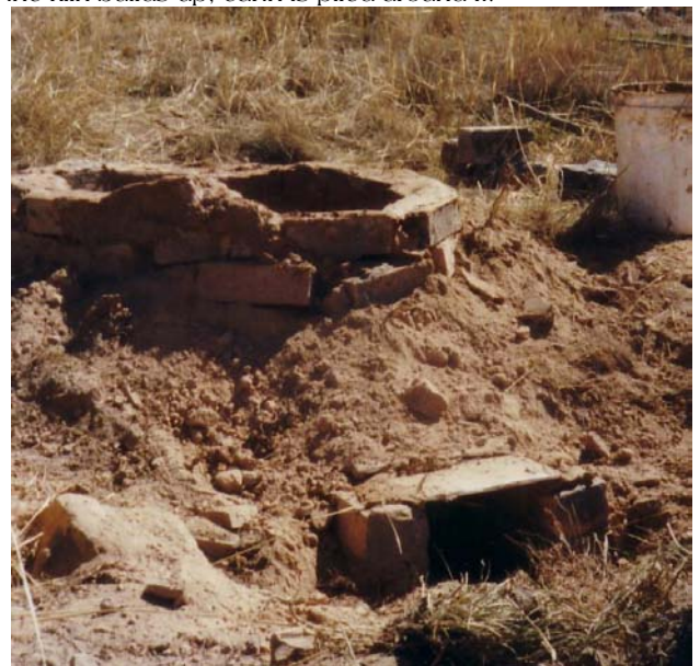
Master Alex the Potter shows how to make a Roman kiln. Below is the kiln further on in construction. Note that as the kiln builds up, earth is piled around it.
